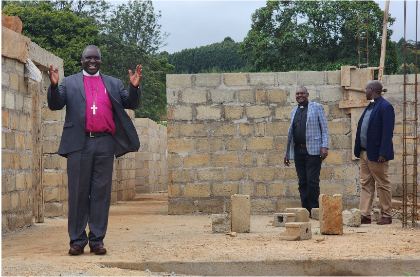
A joyful bishop visits the health clinic's construction site.
