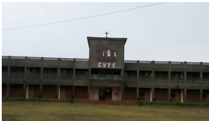
The newly constructed Christian Vocational Training Center was finished in 2016. Funds from the Anglican Relief and Development Fund will equip the school and cover the cost of 100 students' on-campus accommodations.
